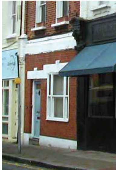
Good example: Victorian language used to give a larger, three sectioned sash window on the ground floor
