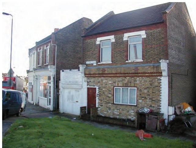
Bad Practice: Shopfront removed
