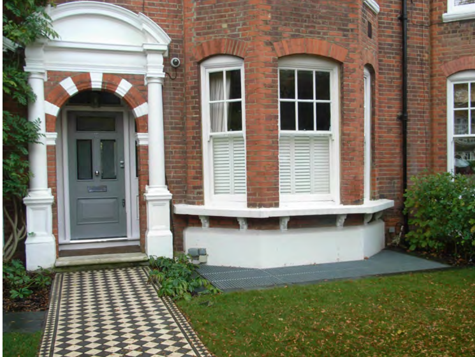
Front lightwell incorporating security grille with over half the depth of the garden retained
